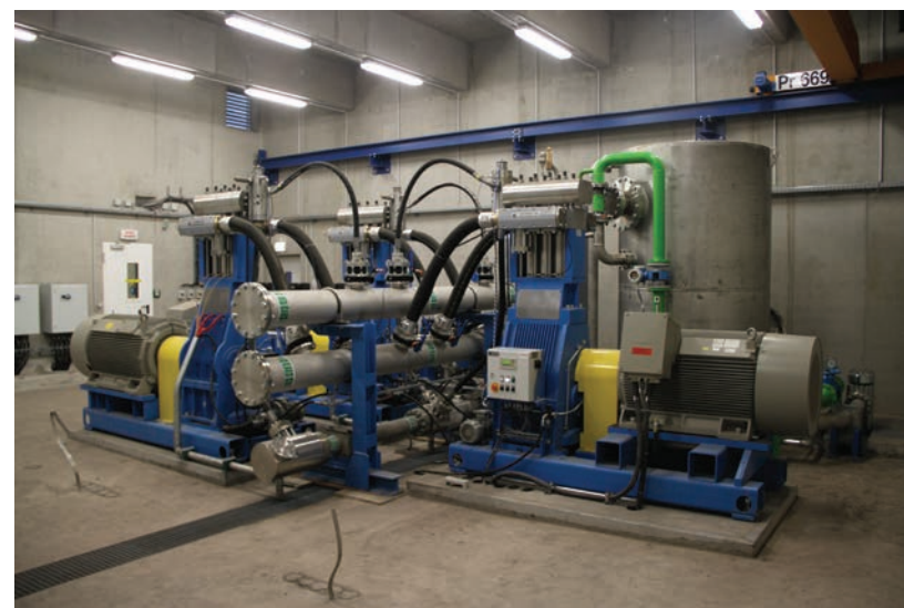
HERMETIK high-pressure pump room with 3 pumps
