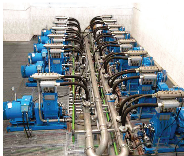
HERMETIK high-pressure pump room with 14 pumps
